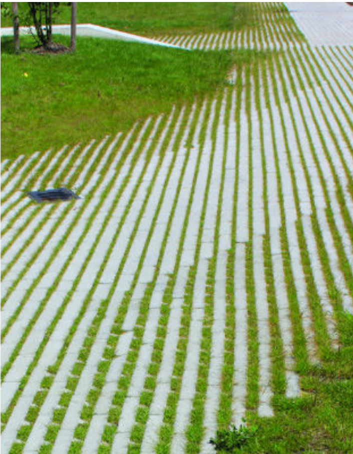
Example of a permeable grasscrete surface
