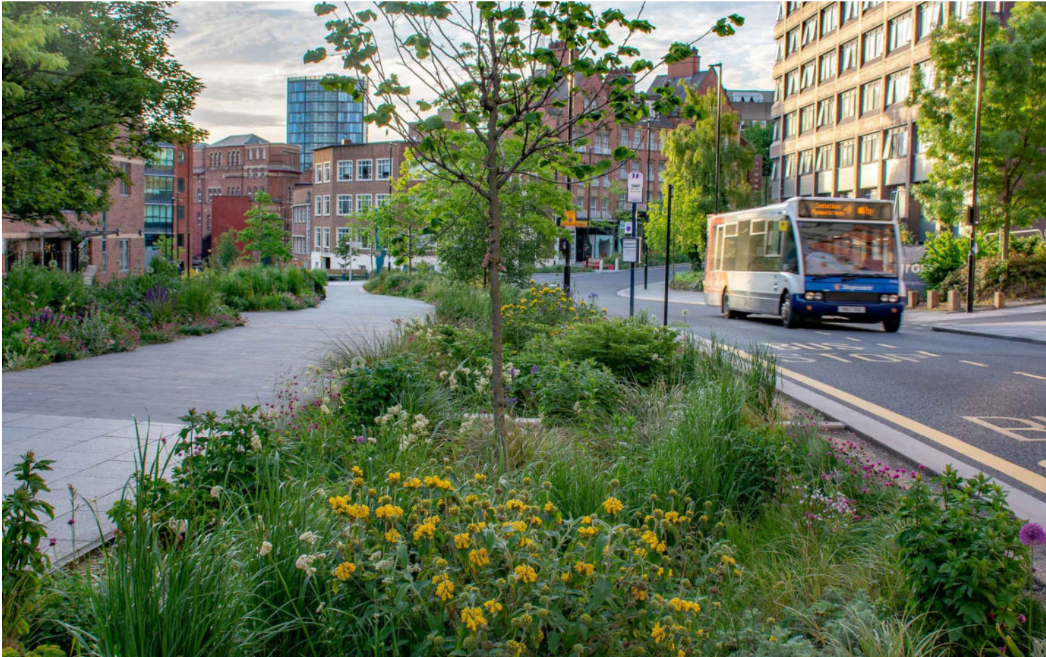
Example of a rain garden with flood tolerant planting species
